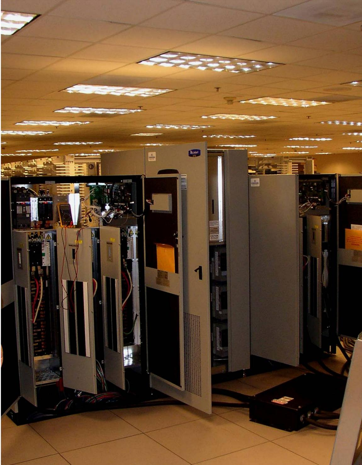
**Figure 1 – Typical PDU in a data center with load bank test being run.**
